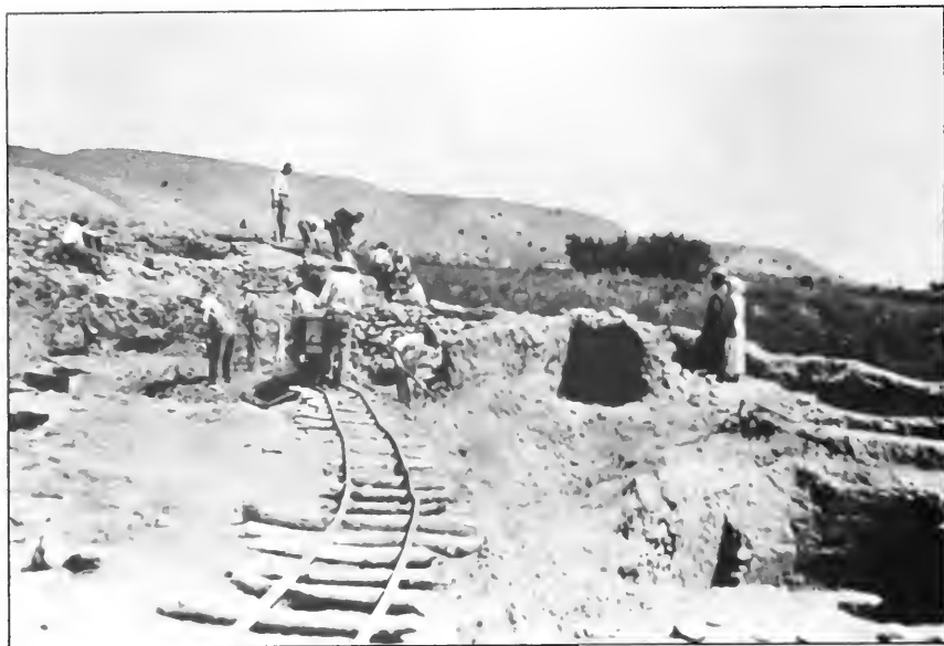
Figure 3.9. East Wing excavations in 1916.
